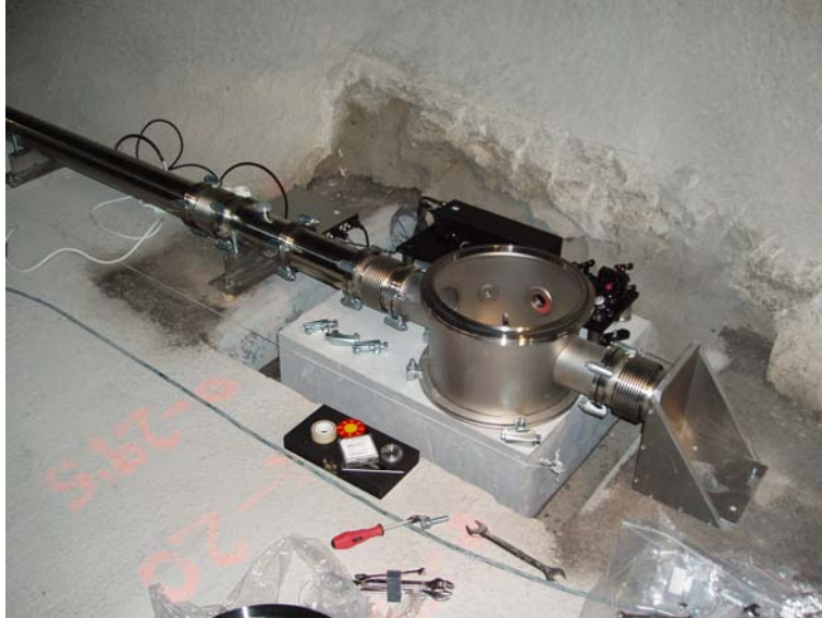
Figure 2: Main plinth in Bypass 16.
